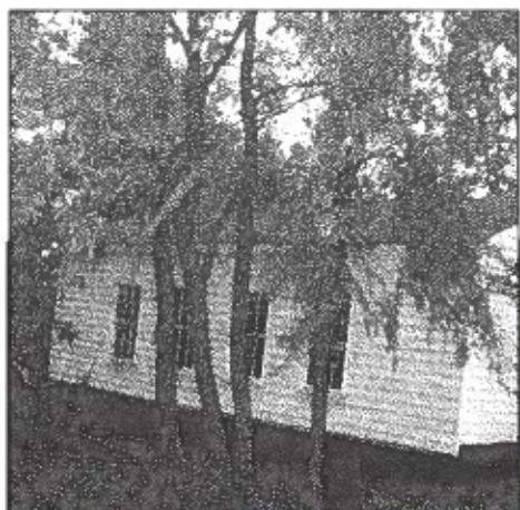
The White Cottage was moved from Myers Park Presbyterian Church and was placed on a platform until the weather improved. PHOTO FROM JLC ARCHIVES
